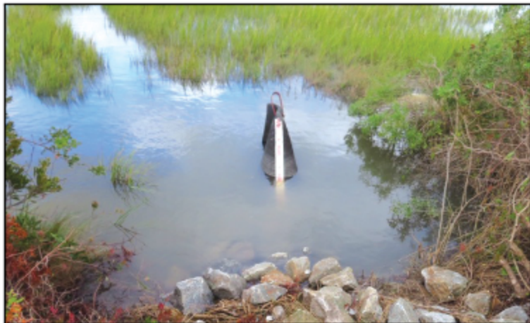
Top of tide gate at high tide October 11
